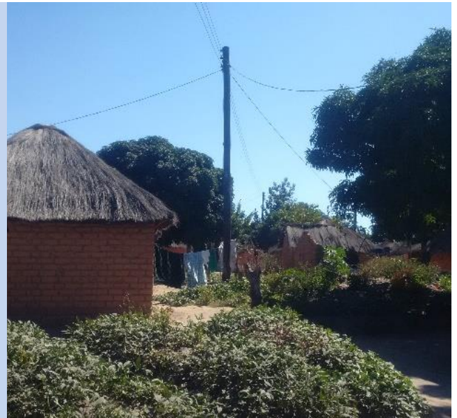
Rural community connected with mini-grid electricity. Over 50% no longer use the electricity mainly due to electricity price
